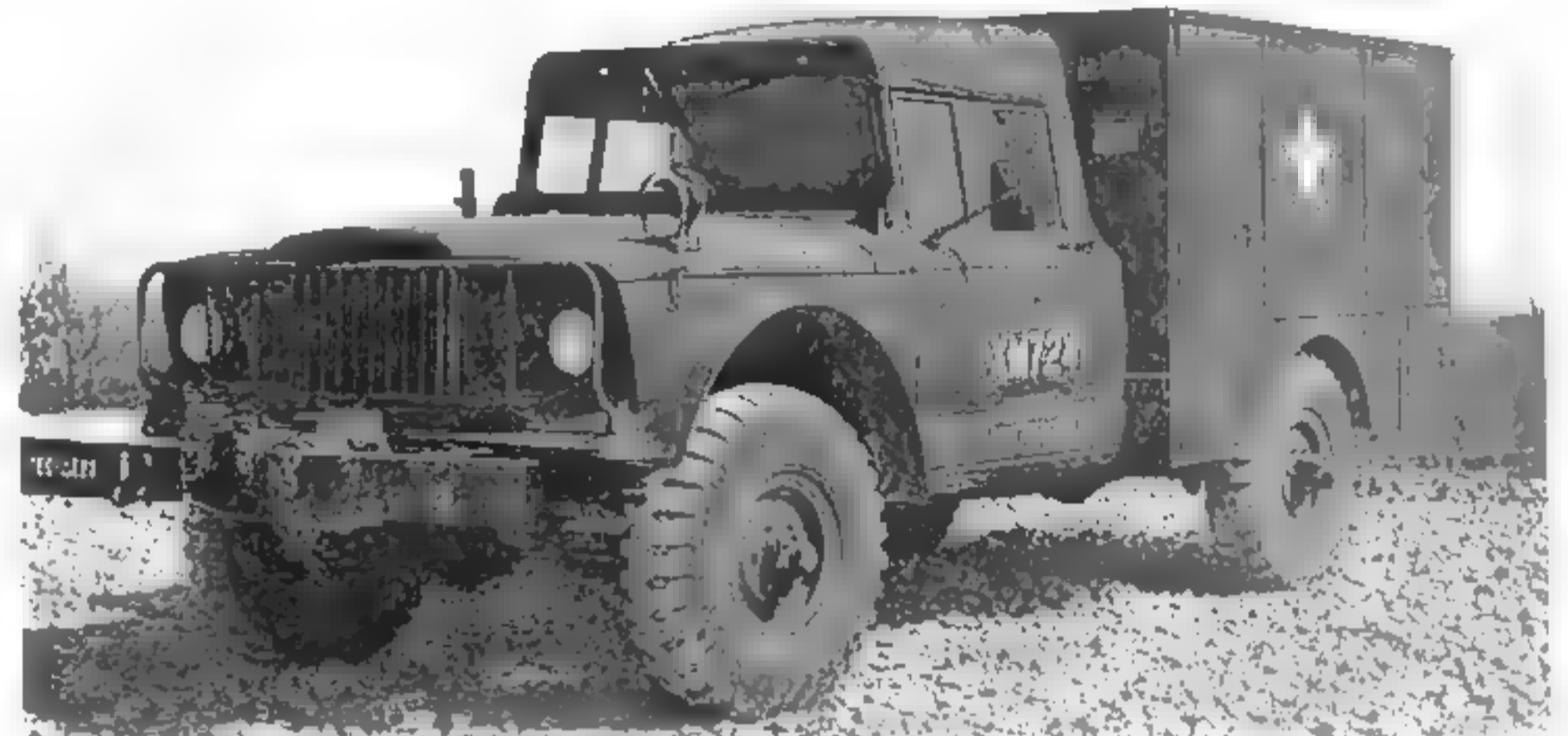
The 6217 contact maintenance truck (above) is often erroneously referred to as an M724. A host of tools and equipment were carried in the compartments, while a large PTO-driven combination welder/generator was mounted inside the bed. (Photo courtesy the Patton Museum)
